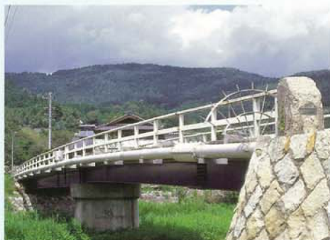
SUS304 200A/100A二重保温管橋梁添架
